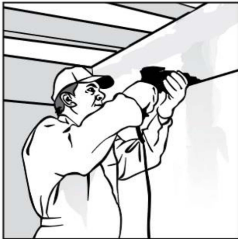
1. Fixing the perimeter L-channel
