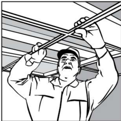
3. Installing the suspended grid
