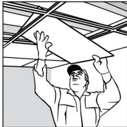
4. Placing the tiles in the grid frames
