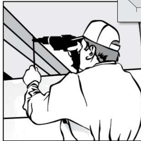
2. Fixing the hangers to the main soffit
